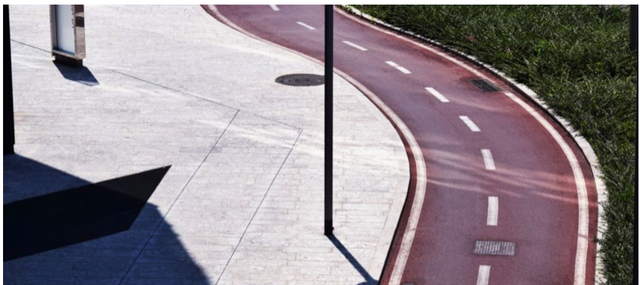
Figure O.2.5: Use different surface materials to demarcate a pathway and define its edge
