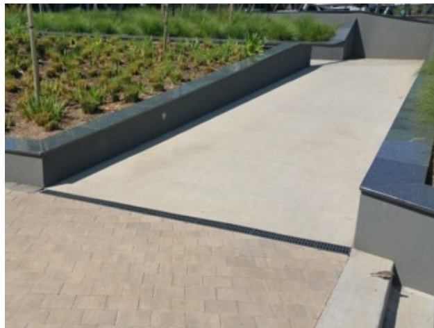
Figure O.2.6: Both stairs and ramps should be provided (L) and ramps should have landings at convenient intervals (R)
