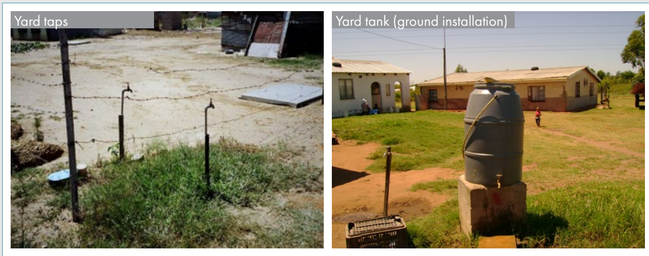
Figure J.6: Examples of private end-user points of supply
