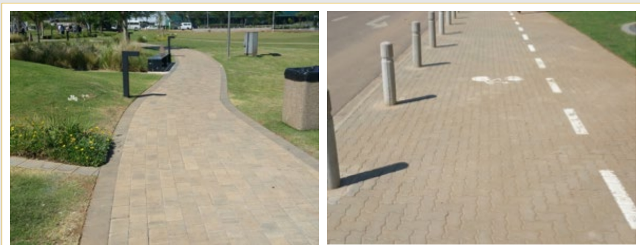
Figure O.2.3: Street furniture should be carefully positioned to maintain a clear pathway
