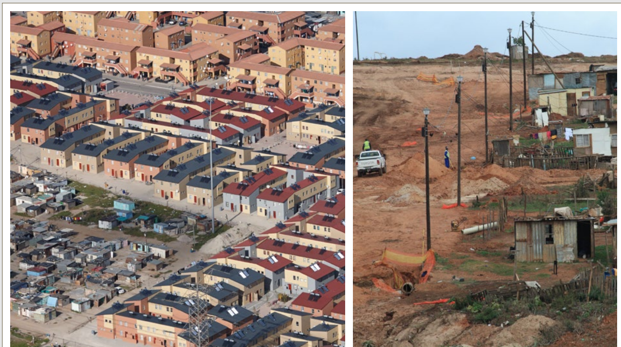
Figure D.4: Examples of informal settlement upgrading
