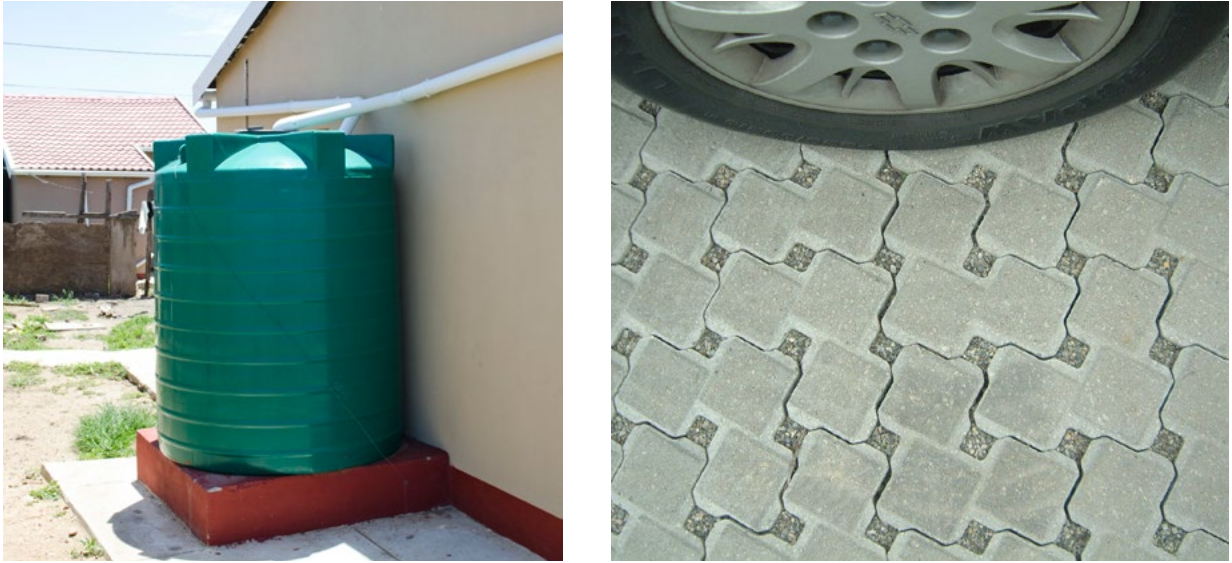
Figure L.6: A rainwater harvesting system (L) and permeable pavement (R)
