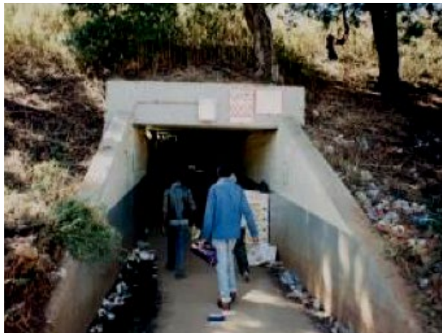
Figure O.1.6: Once someone has entered this subway, opportunities to escape an offender are limited
