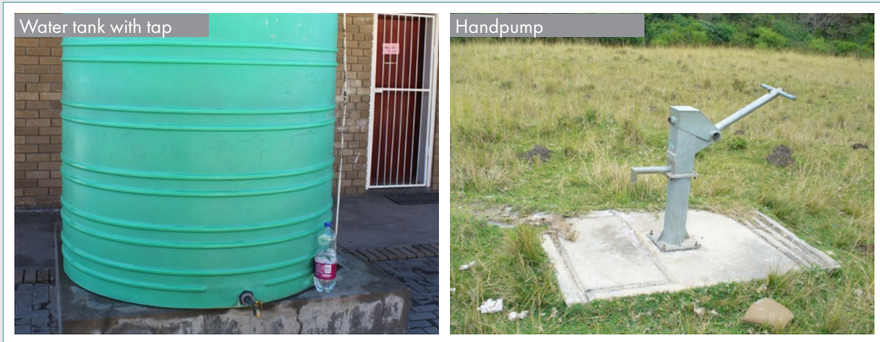
Figure J.5: Examples of public (communal) end-user points of supply
