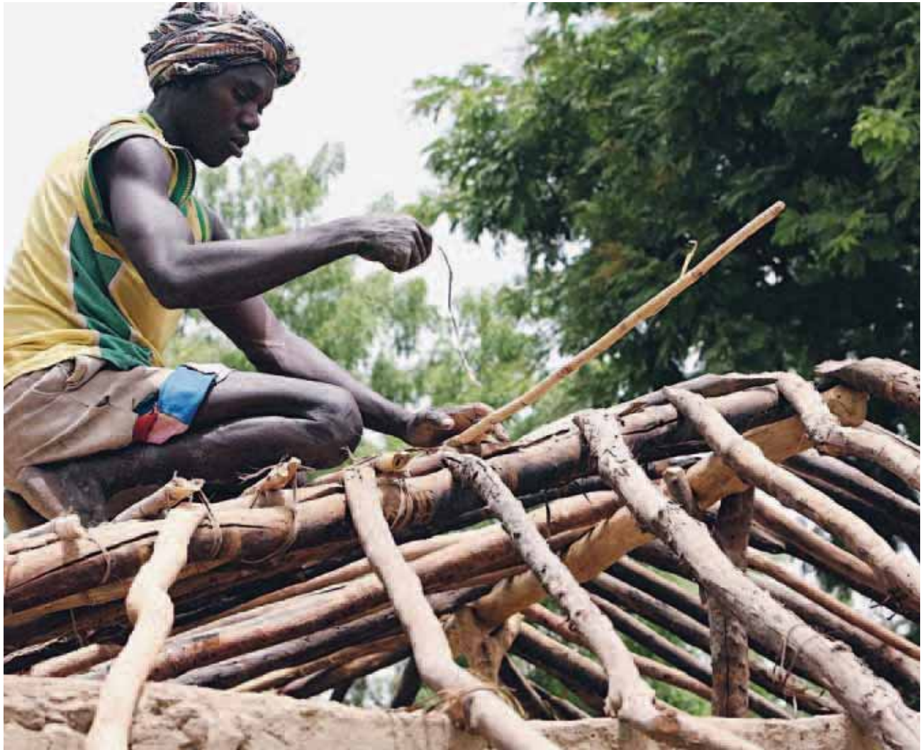
▲ Roof construction, Central African Republic. ©Anthony Morland/IRIN
