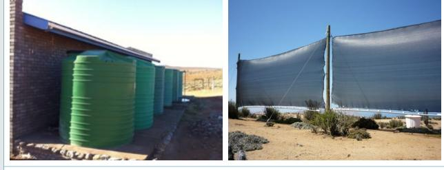
Figure J.10: Rainwater harvesting (L) and fog harvesting (R)
