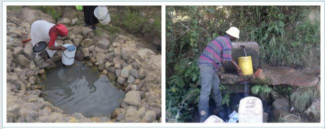
Figure J.8: An open spring (L) and a protected spring (R)
