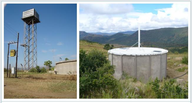
Figure J.3: Examples of concrete and metal reservoirs (L) and a concrete reservoir (R)
