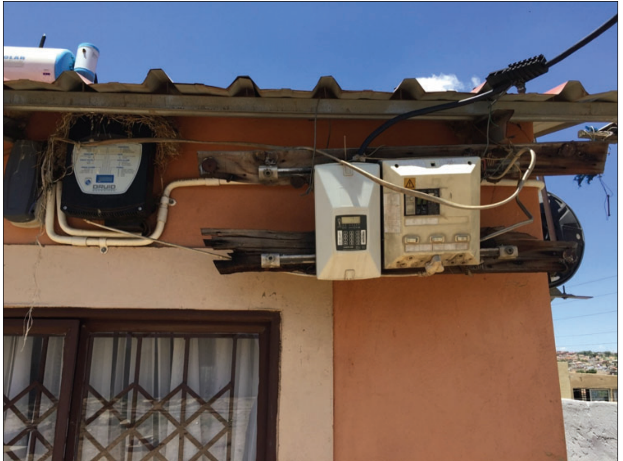
Figure 12: A unit with the electric box installed outside the house. Source: Authors' images
