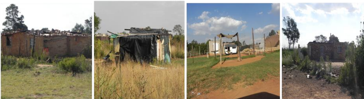
Figure 4: Pictures representing various housing typologies in the Springvalley area
