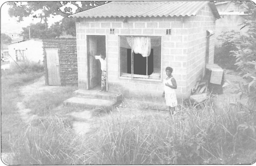
Inanda Newtown: two-room core house
