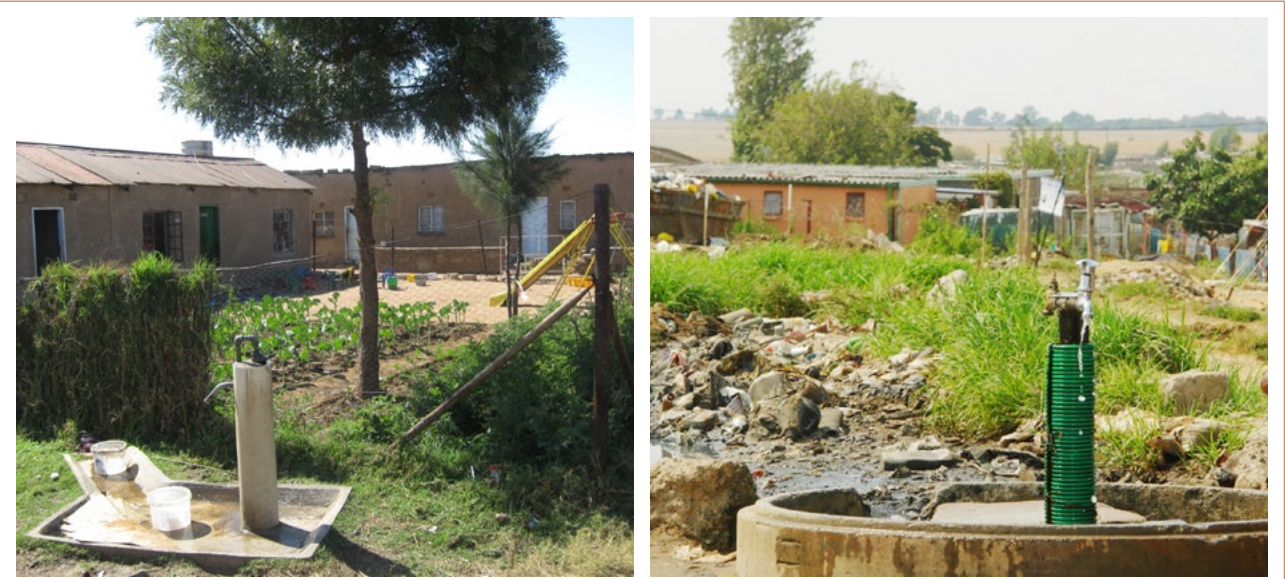
Figure L.3: Excess water at a communal standpipe redirected for garden use (L) and excess water causing erosion (R)
