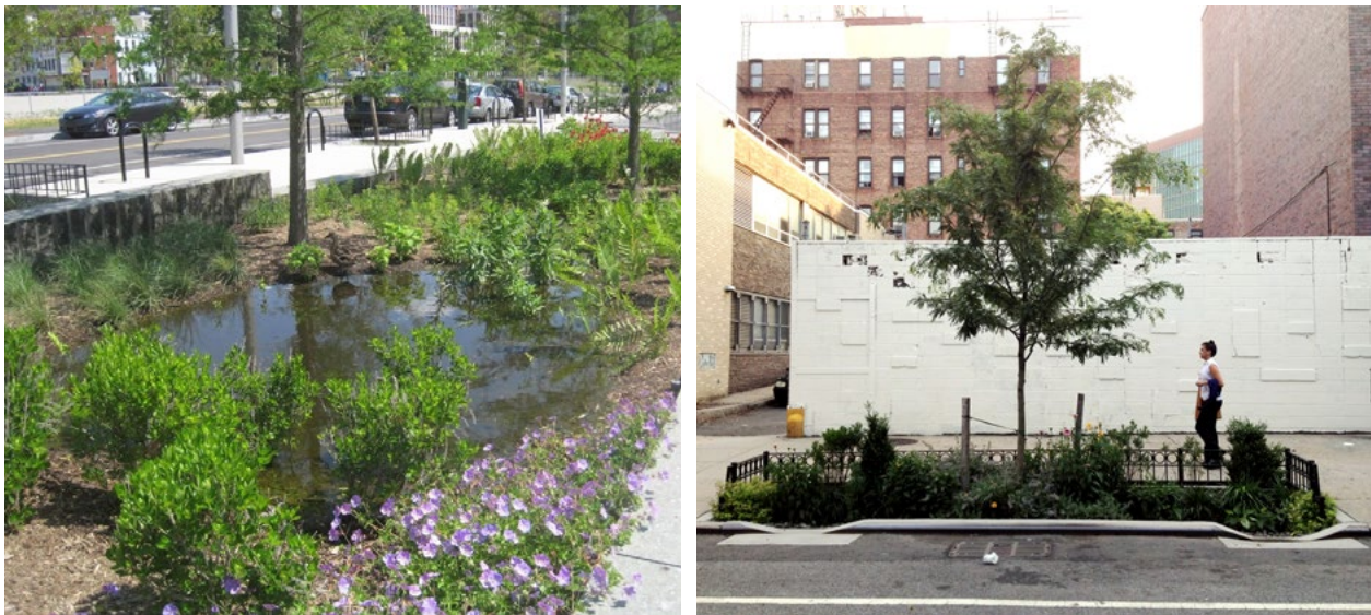
Figure L.7: Examples of a rain garden (L) and a bioswale (R)
