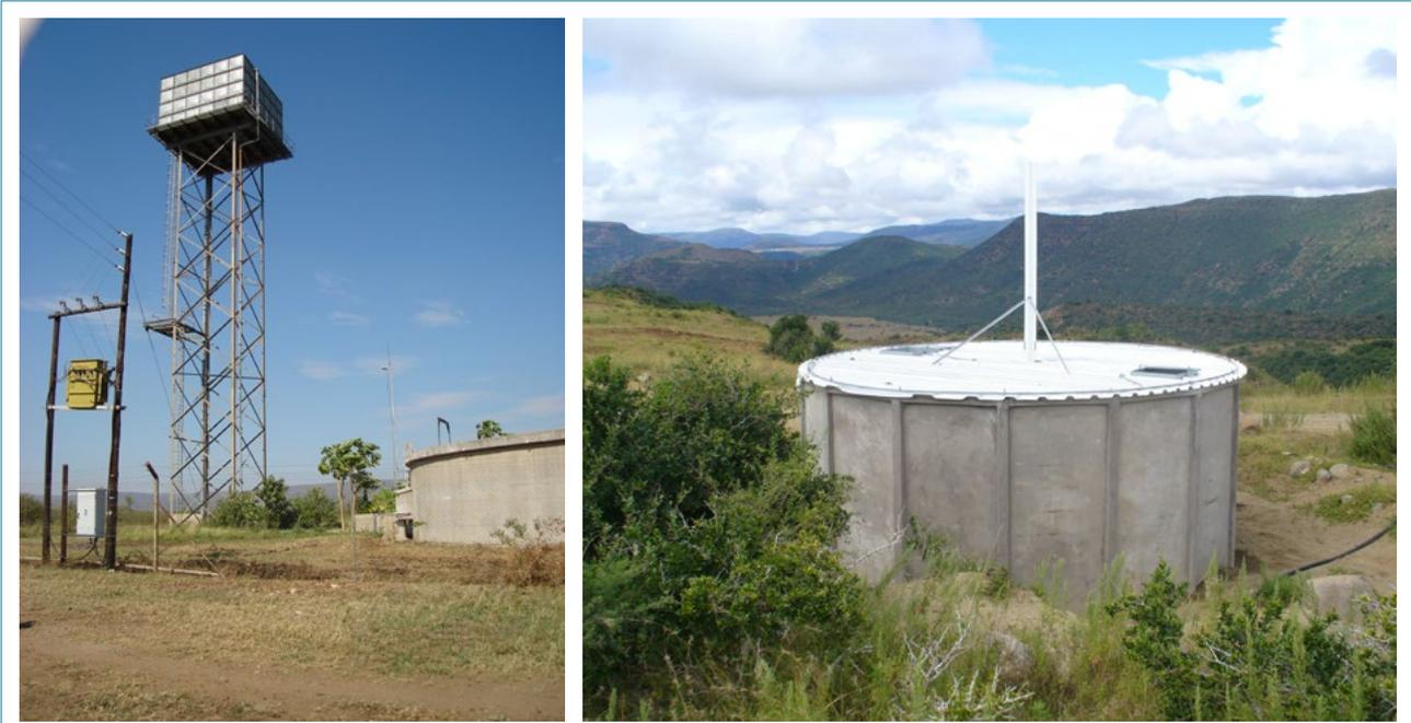
Figure J.3: Examples of concrete and metal reservoirs (L) and a concrete reservoir (R)
