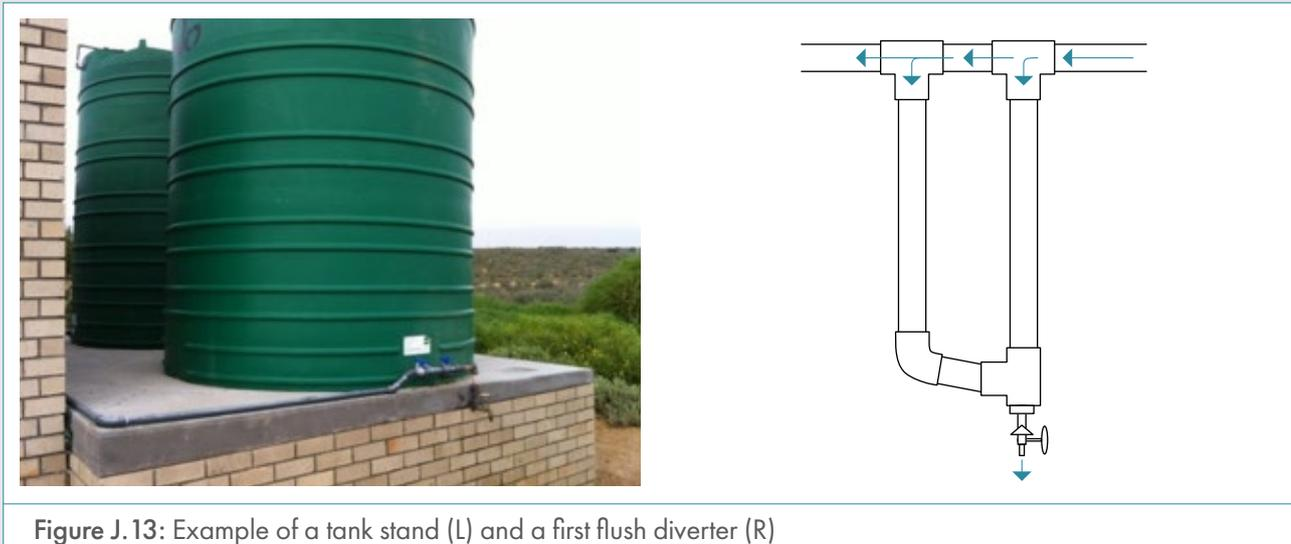
Figure J.13: Example of a tank stand (L) and a first flush diverter (R)
