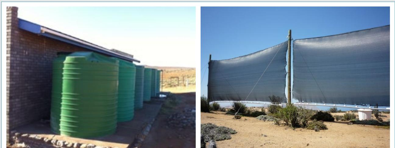
Figure J.10: Rainwater harvesting (L) and fog harvesting (R)
