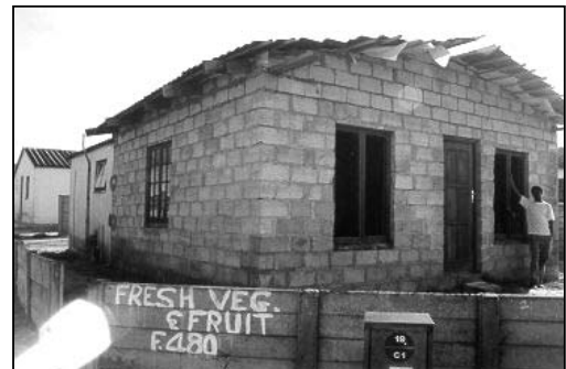
Photo 6-21: Corner shop being built
