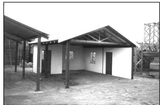
Photo 2-1: South African version of a roof house, Durban
