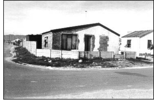
Photo 6-13: Khayelitsha windows, door and roof alterations
