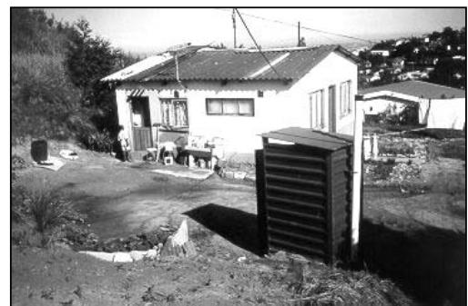
Photo 6-15: Inanda pit latrine
