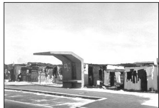
Photo 4-13: Bus stop on boundary street
