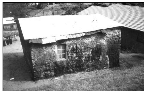
Photo 6-3: Lodging or family accommodation? Inanda backyard room
