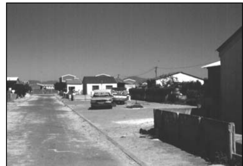
Photo 4-15: Widening of roads at mid-block
