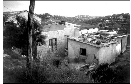
Photo 6-6: Inanda concrete block extension
