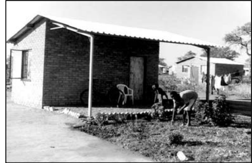
Photo 2-3: Half roof house, half core house, Giyani (source: DoH)
