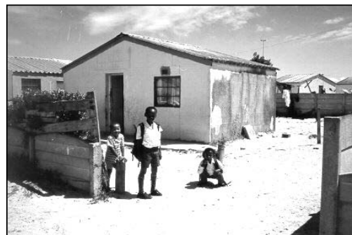
Photo 8-10: House where an adjoining shack burnt down, Khayelitsha
