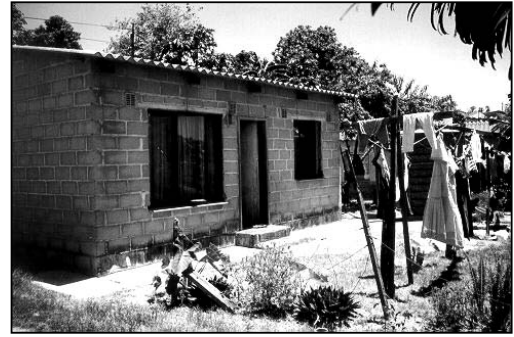
Photo 5-2: Inanda Newtown four room house
