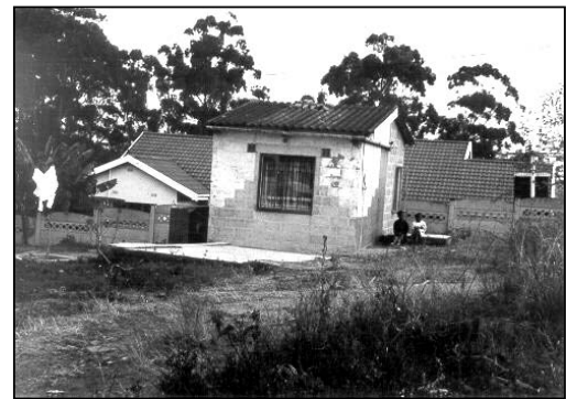
Photo 4-12: Two room Urban Foundation show house
