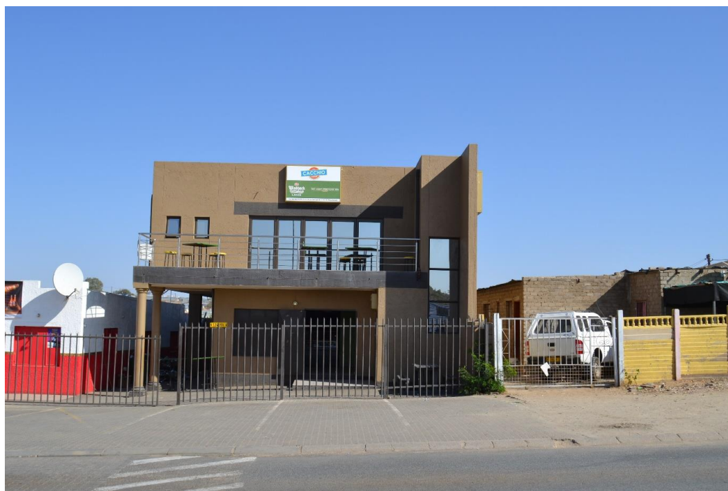
Figure 6.7: Vertical renovation, Eveline Street
