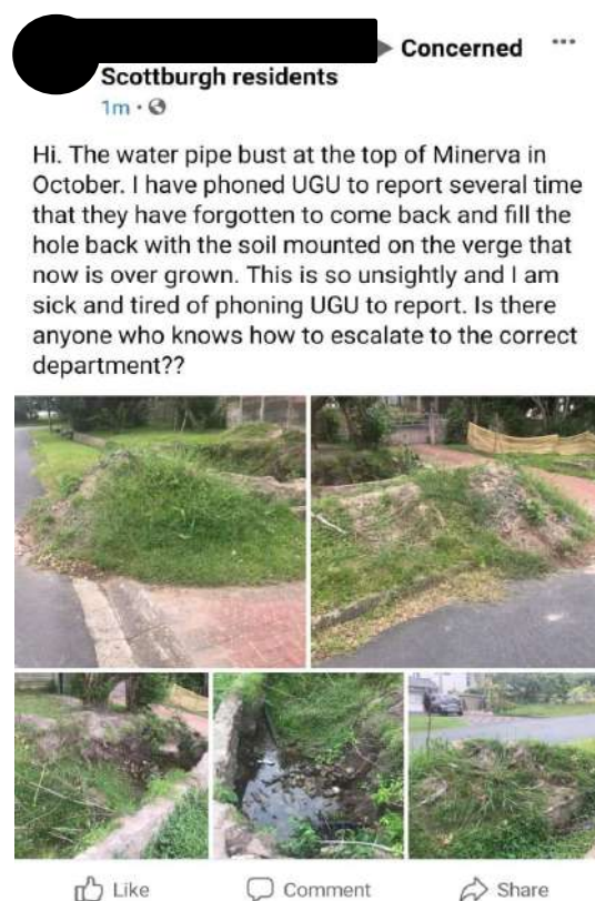
Photo 6.5. Example of poor infrastructure maintenance
