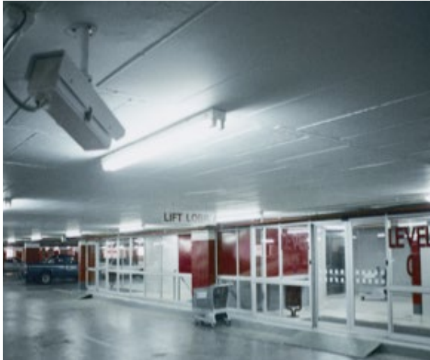
Figure O.1.1: The glass lobby increases visibility and the CCTV camera provides additional surveillance
