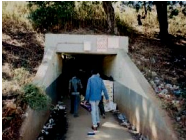
Figure O.1.6: Once someone has entered this subway, opportunities to escape an offender are limited
