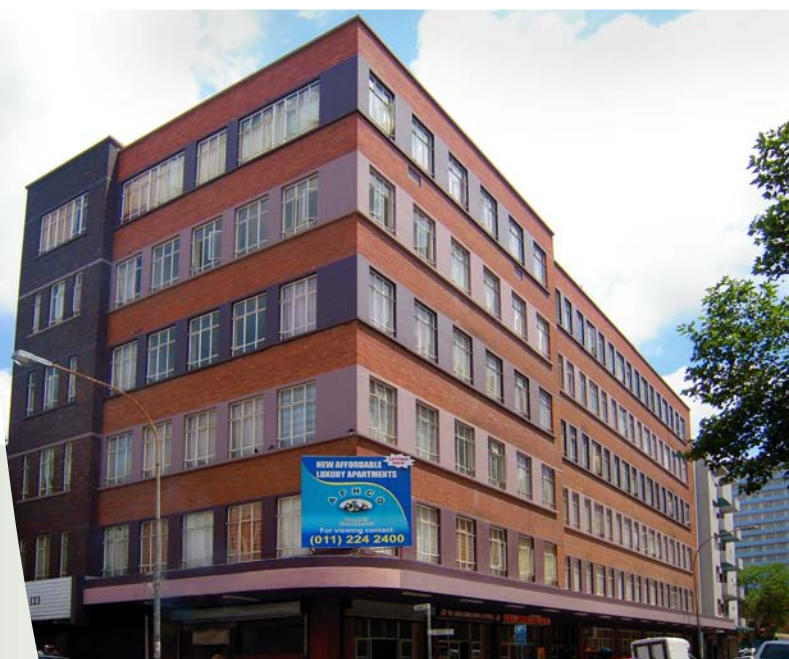
Private sector affordable inner city housing within the Johannesburg Urban Development Zone
