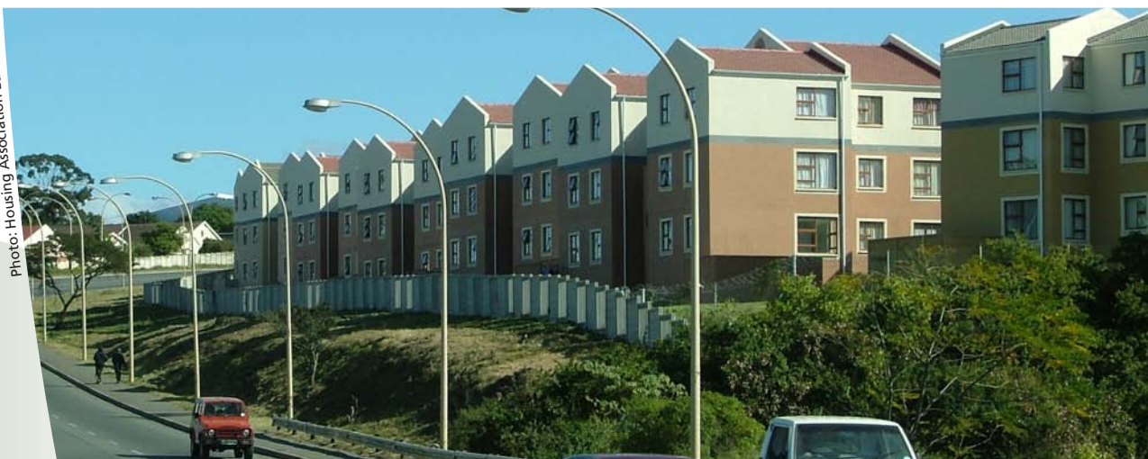
Social housing in East London – a form of state intervention through subsidies
