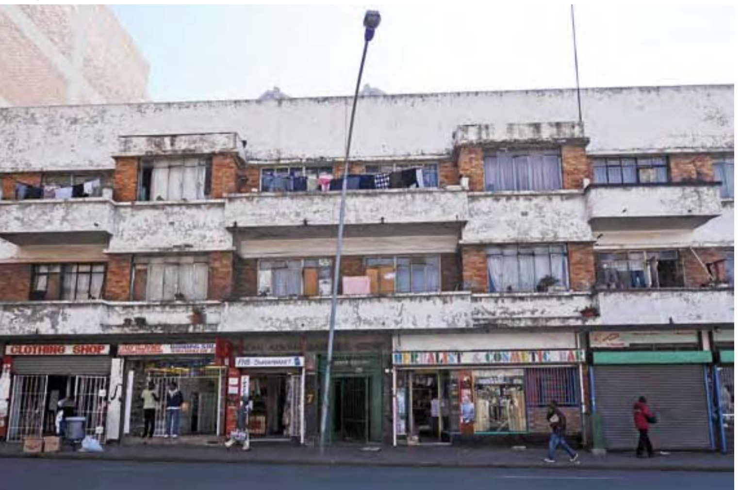
A residential building and commercial premises in the Doornfontein precinct.
