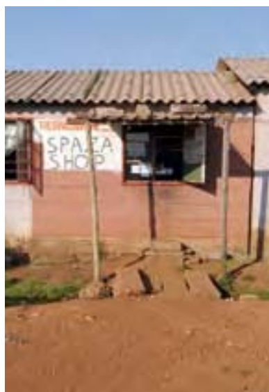
A spaza shop built on to an informal dwelling in Diepkloof.
