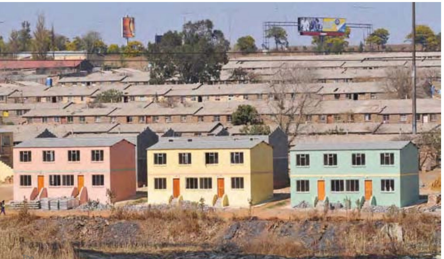
The Community Residential Unit development juxtaposed with the old hostels in Diepkloof.
