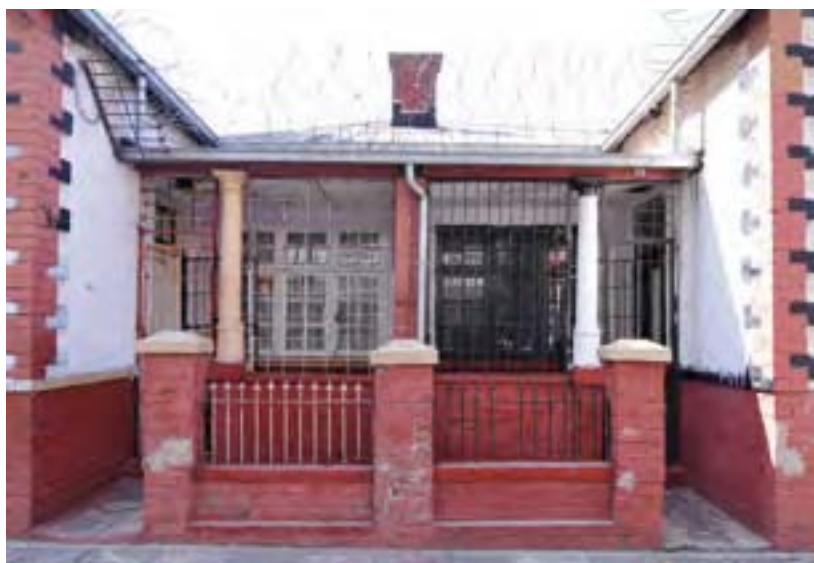
Original Doornfontein house made secure against the criminality in the area.
