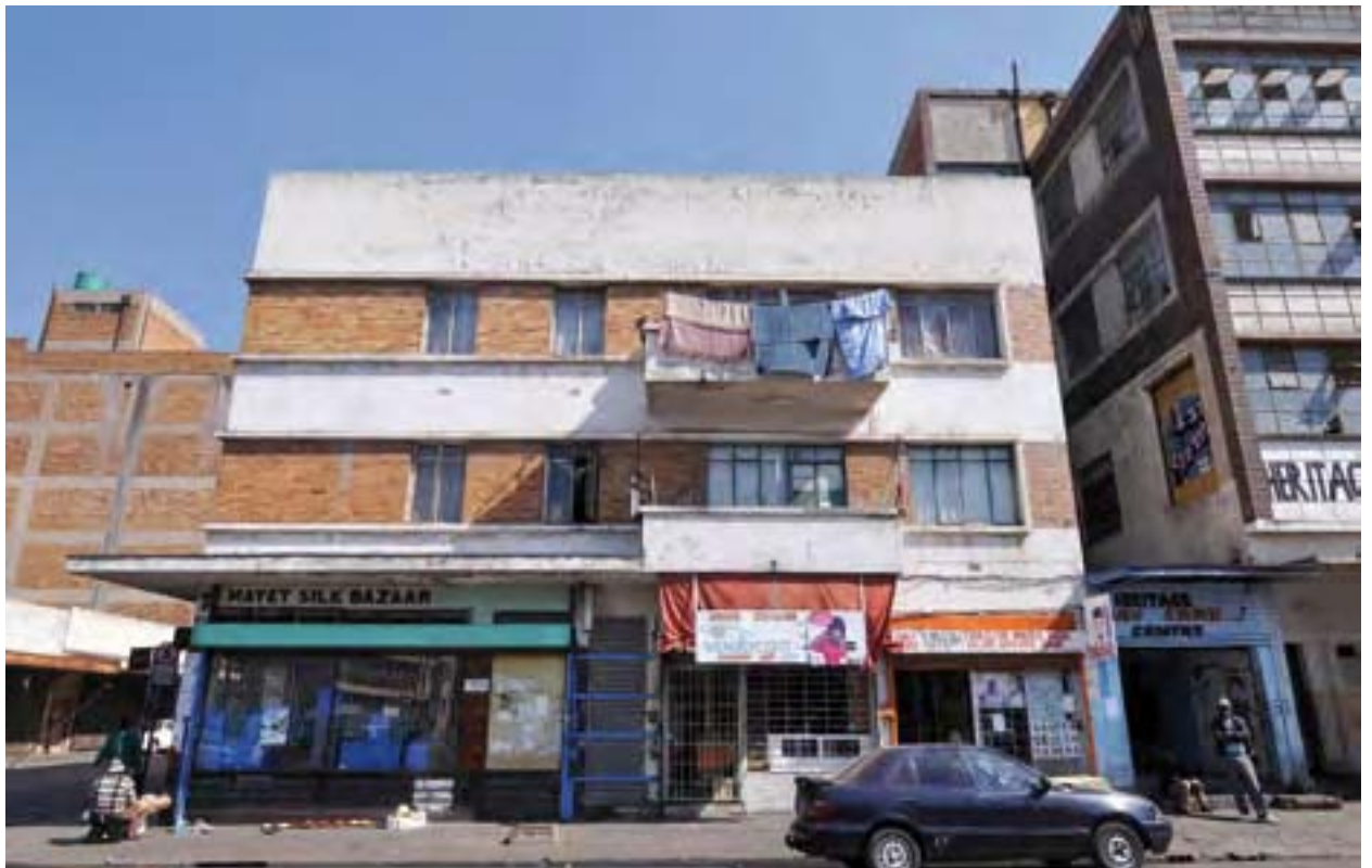
A degraded residential building and downstairs retailers' premises in Doornfontein.
