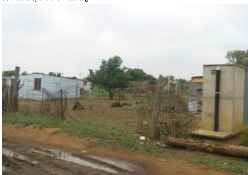
Figure 5: A VIP toilet installed during Regularisation
