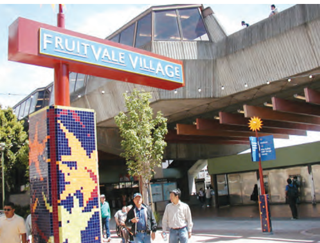
Fruitvale Village BART station
