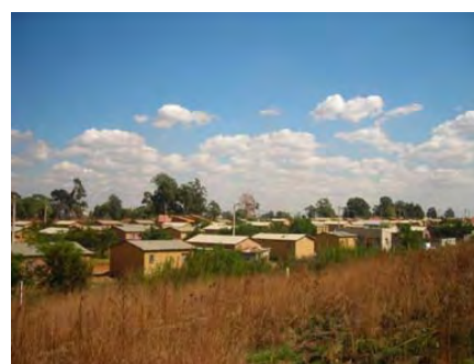
Kingsway RDP housing (established 1989)
